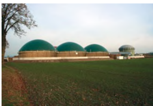
Waste digestion plant (1 MW el ) with an input of 24,000 t per year
