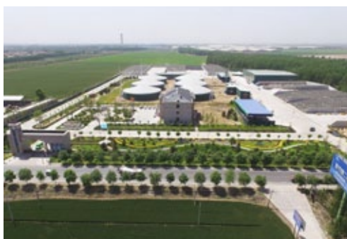
The biogas and biomethane plant in Dingzhou, China produces 400 Nm 3 per hour of biomethane for the transport sector
