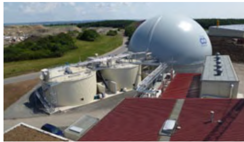
Wet fermentation system operated by the "Fitec"-process of the Finsterwalder Umwelttechnik GmbH & Co. KG, Rothmühle AD Schweinfurt Germany
