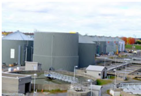
LIPP digesters and process tanks at St. Hyacinthe, Canada – producing biogas from sludge and biowaste.
