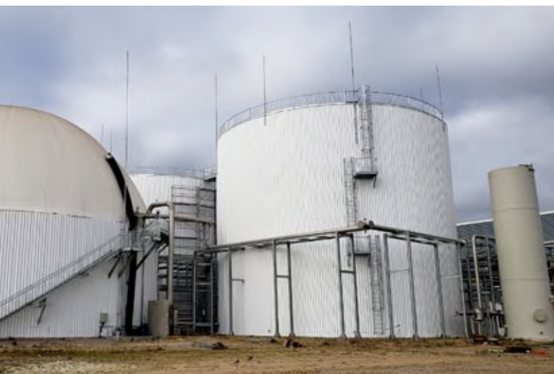
Gasholder, digester and desulphurisation plant
