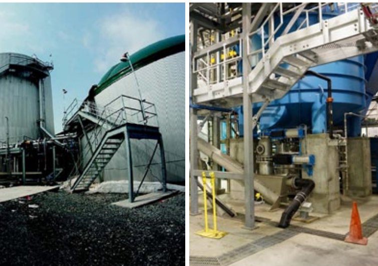
Digesters (left) and BTA Waste Pulper (right). Varennes, Canada.
