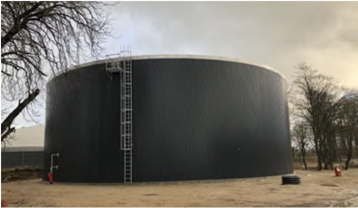
Stainless steel digester with insulated stainless steel roof for glycerin
