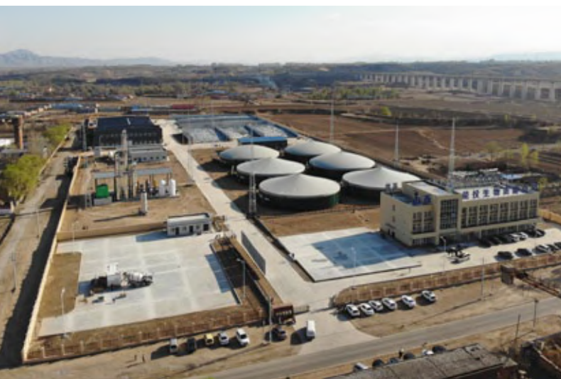
The biogas plant in Shanxi province produces 37,680 m³/d from energy crops and animal by-products.
